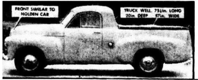
FIRST picture of the new Holden seven-cwt, utility—the first utility truck to be made completely in Australia.
